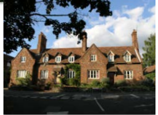
Dairy & Hill cottages
