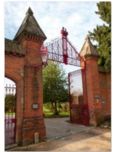
N Lodge gates & piers
