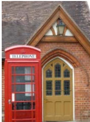
K6 telephone box
